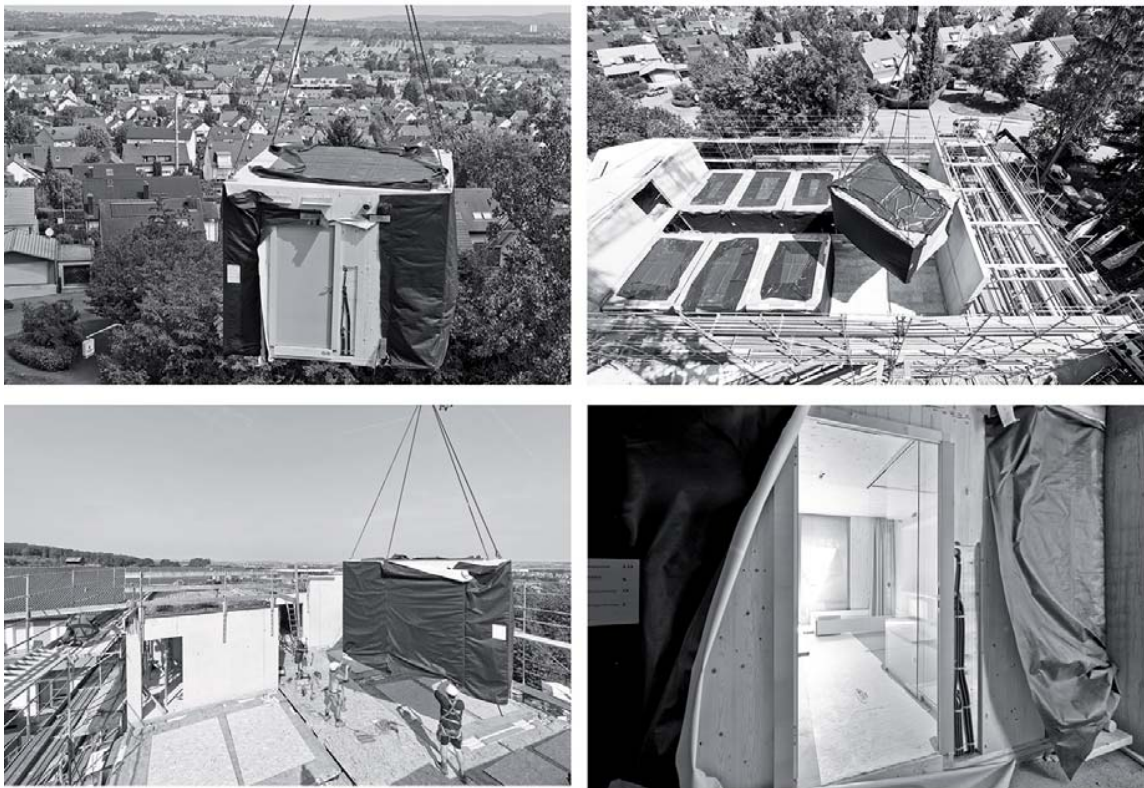
Fig 3 a – d Assembly and Installation Sequences of CLT-Room Modules
